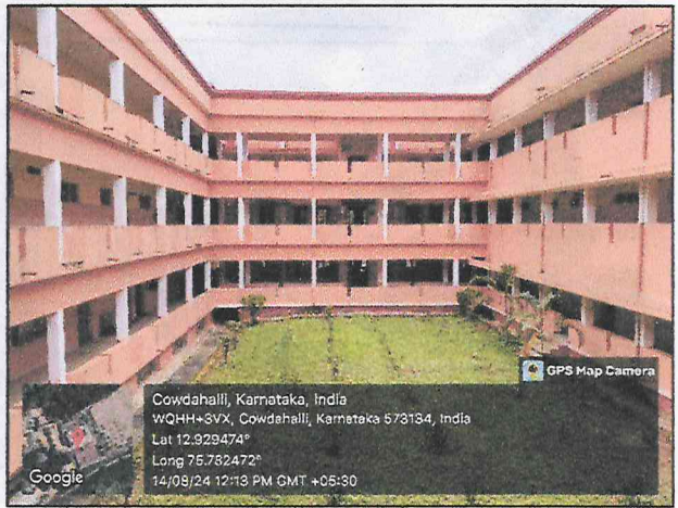
Building Interior View
